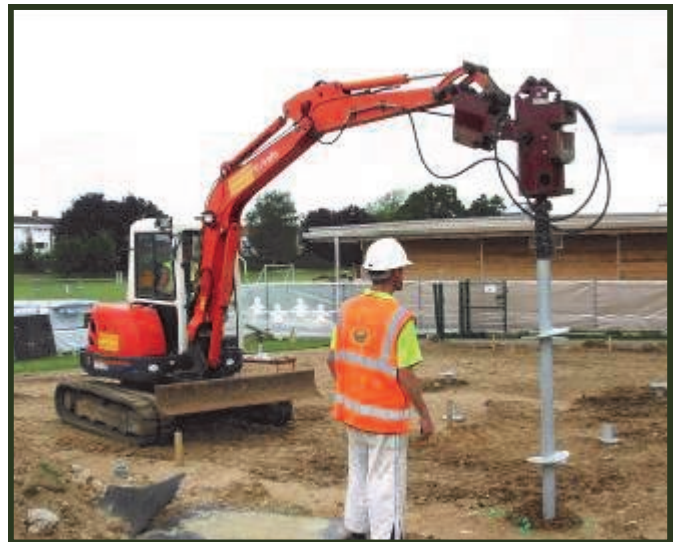
A Screw Pile being installed on a Cabinco site
